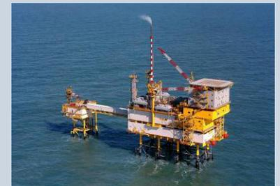
K12-B platform in the Dutch sector of the North Sea where CO<sub>2</sub> is being injected into the same reservoir from which it was extracted
