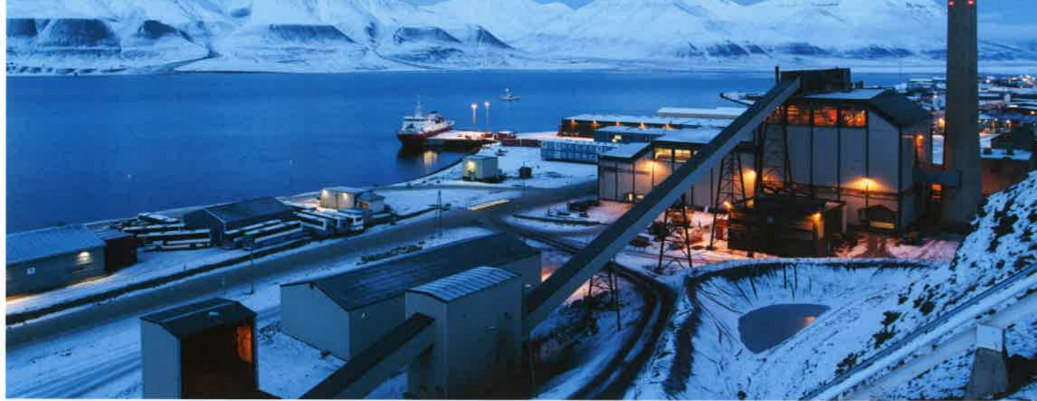
Today's coal-fired power station in Longyearbyen could be replaced by a plant in Adventdalen equipped for CCS.
